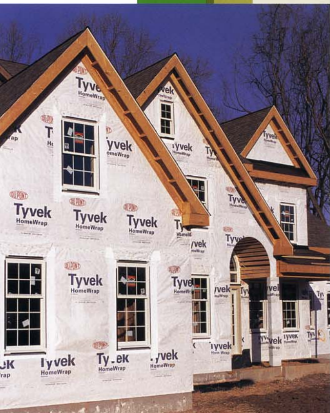
DuPont™ Tyvek® provides a weather-resistant barrier that helps seal the building envelope for more energy efficient, healthier homes in accordance with the ENERGY STAR® Home Sealing™ program.
